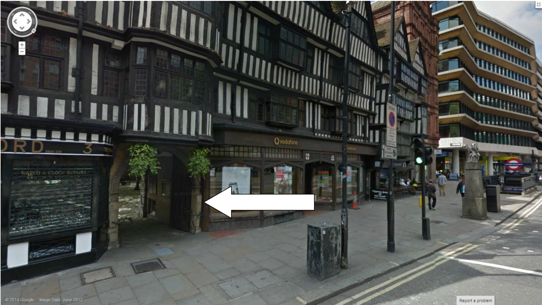
ENTRANCE TO STAPLE INN BUILDINGS (PASSAGEWAY BETWEEN N.3 & VODAFONE SHOP)
